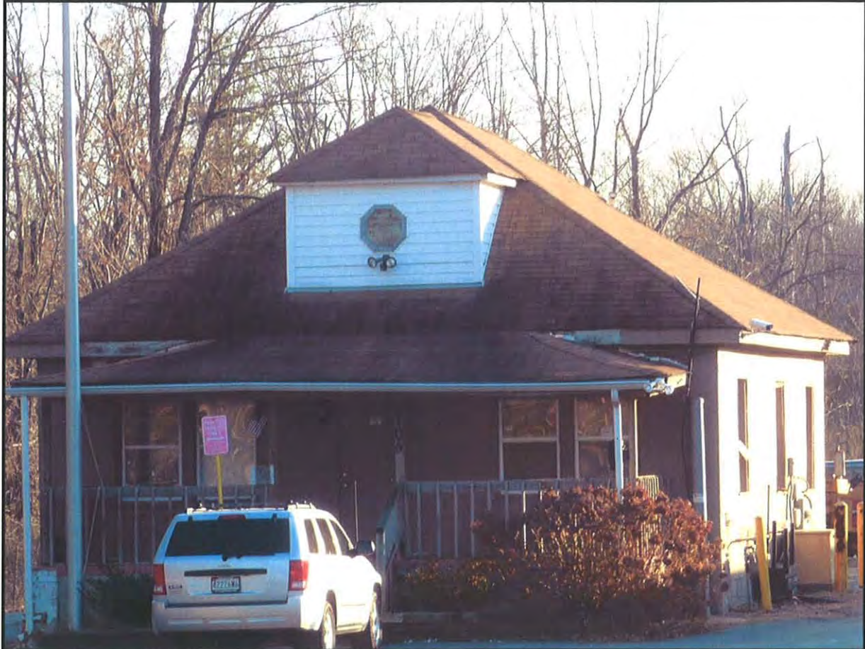
Photograph 1: View of 8705 Westphalia Road, looking south at main elevation. Note modern porch and balustrade, as well as heavily altered dormer. The residence has been converted into offices for the business in this location.
