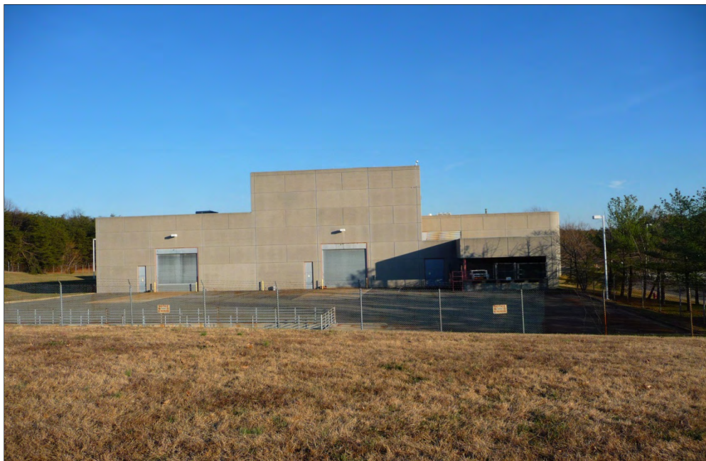
Plate 8: Alternative B, project site showing shop constructed in the 1980s
