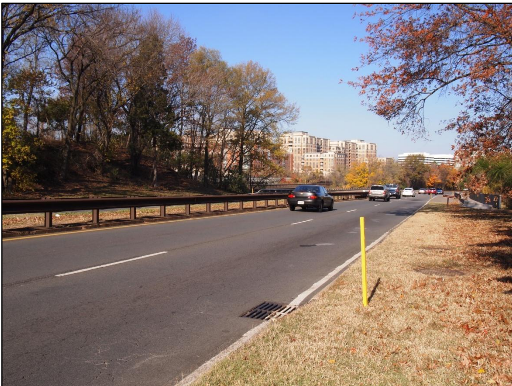
Plate 10: View northbound on the MVMH/PNCR approaching Four Mile Run. Vegetation on west side of MVMH/PNCR would be removed as part of construction of the proposed Build Alternative D.
