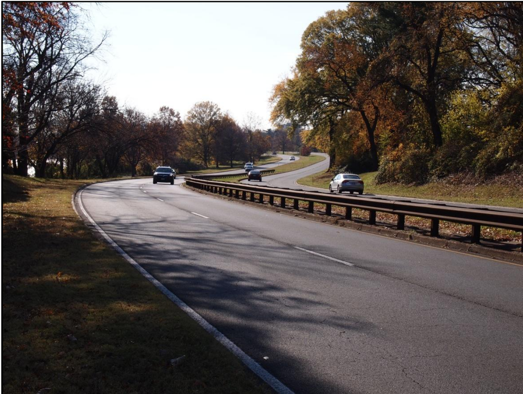
Plate 3: View south on the MVMH/PNCR from the northern end of APE.
