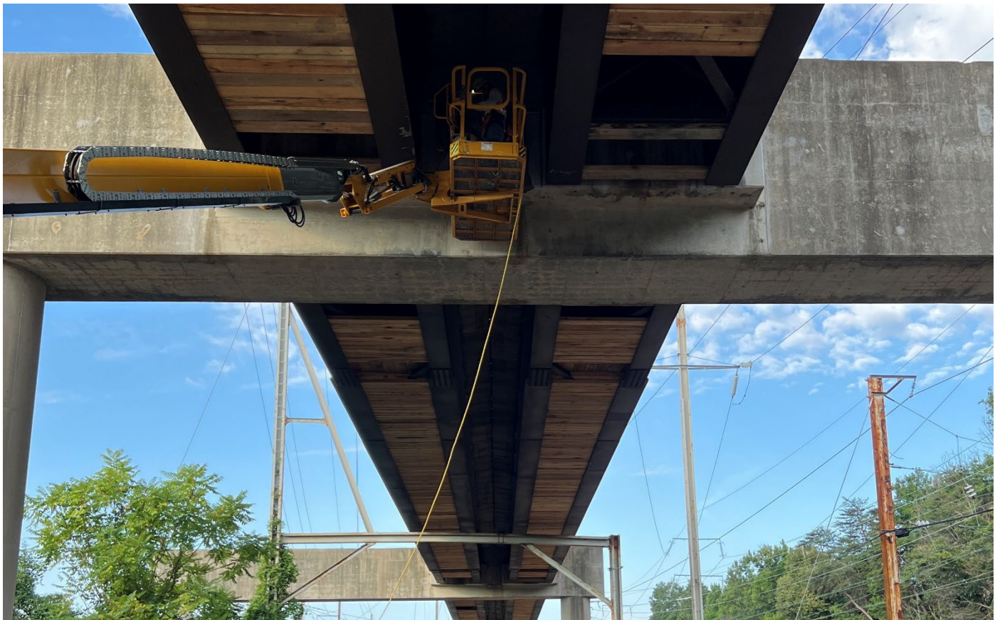
Metro’s Platform Improvement Projects FY2025 constrained funding may limit proactive system investments
