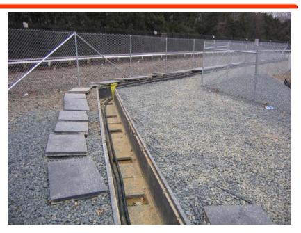
• New MCM traction power cable alongside moisture damaged cable, Traction power cable installation at West Falls Church Station
