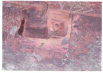
• Moisture and stray current damaged track fasteners
