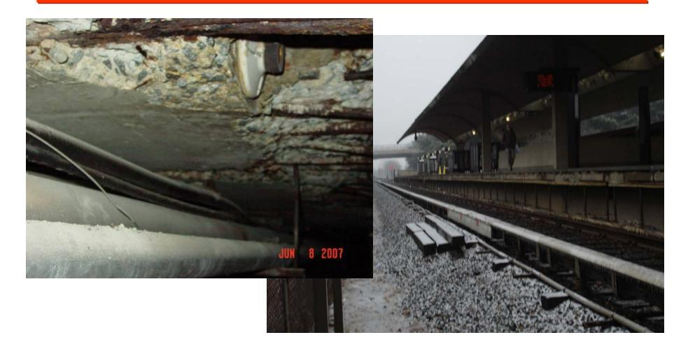
Deterioration of Shady Grove Station platform slab structural concrete
