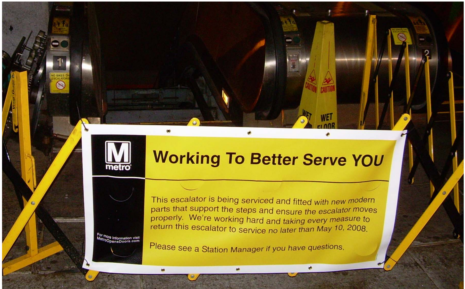
Virginia Square Escalator – Major Repair
