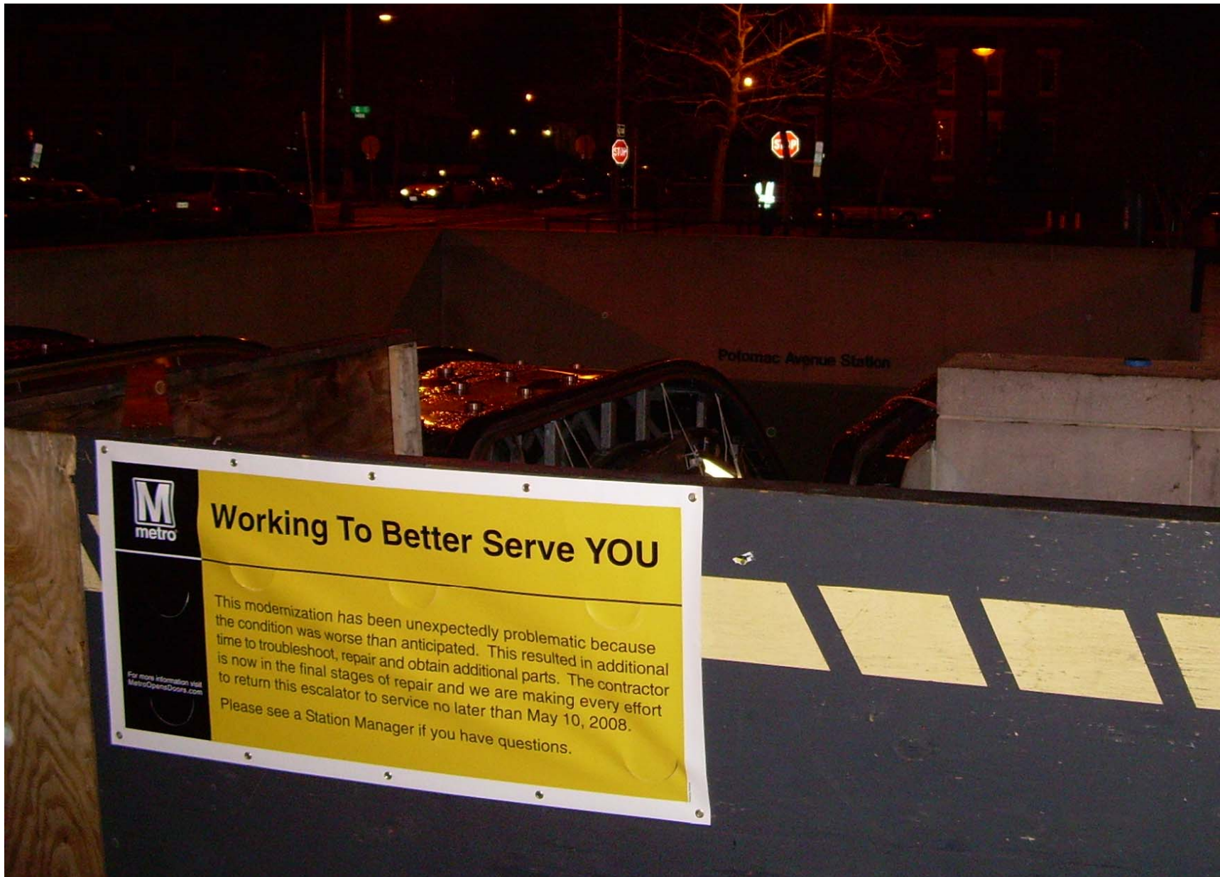
Potomac Avenue Escalator – Rehab/modernization
