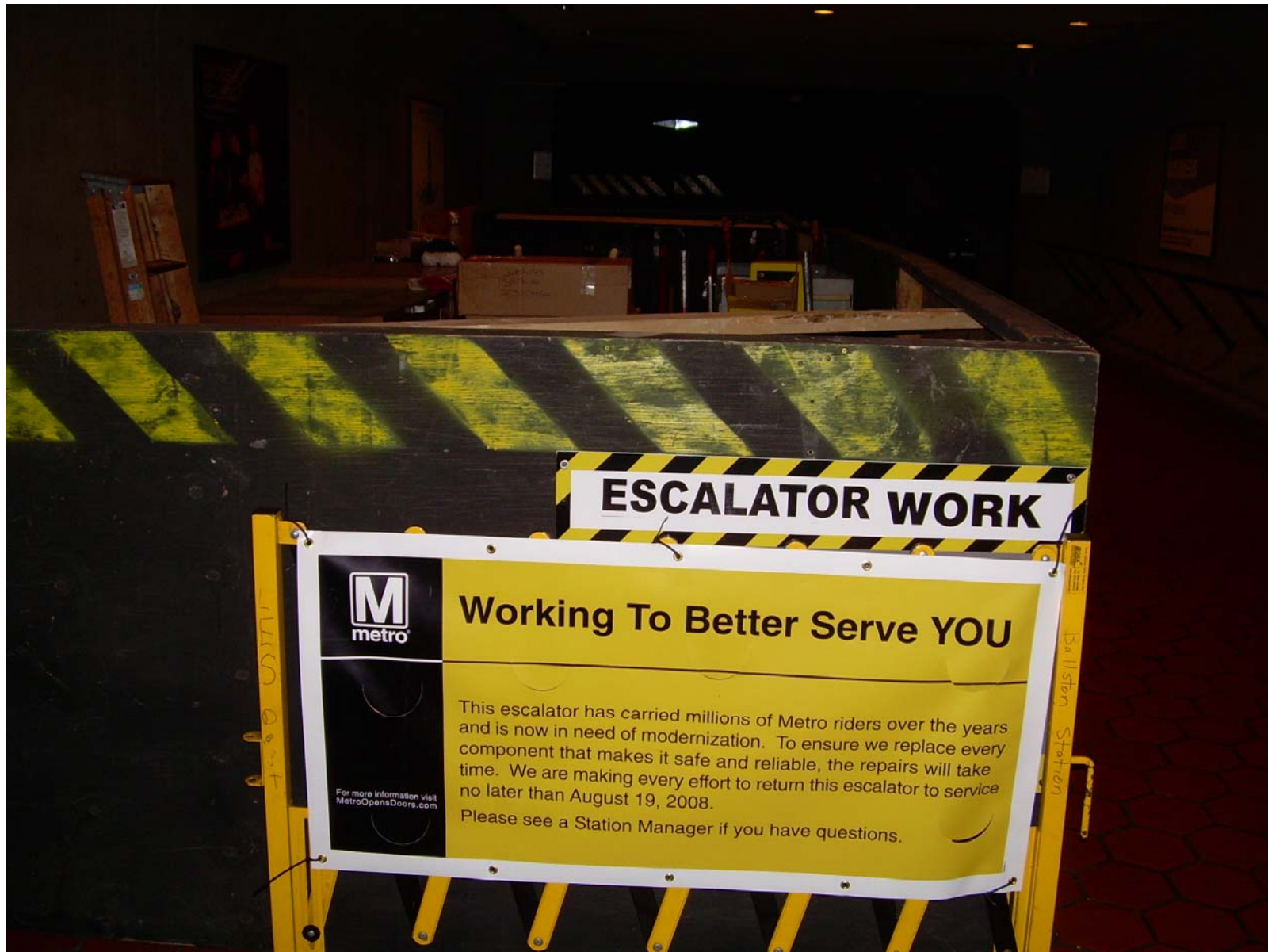
Ballston Escalator – Rehab/modernization
