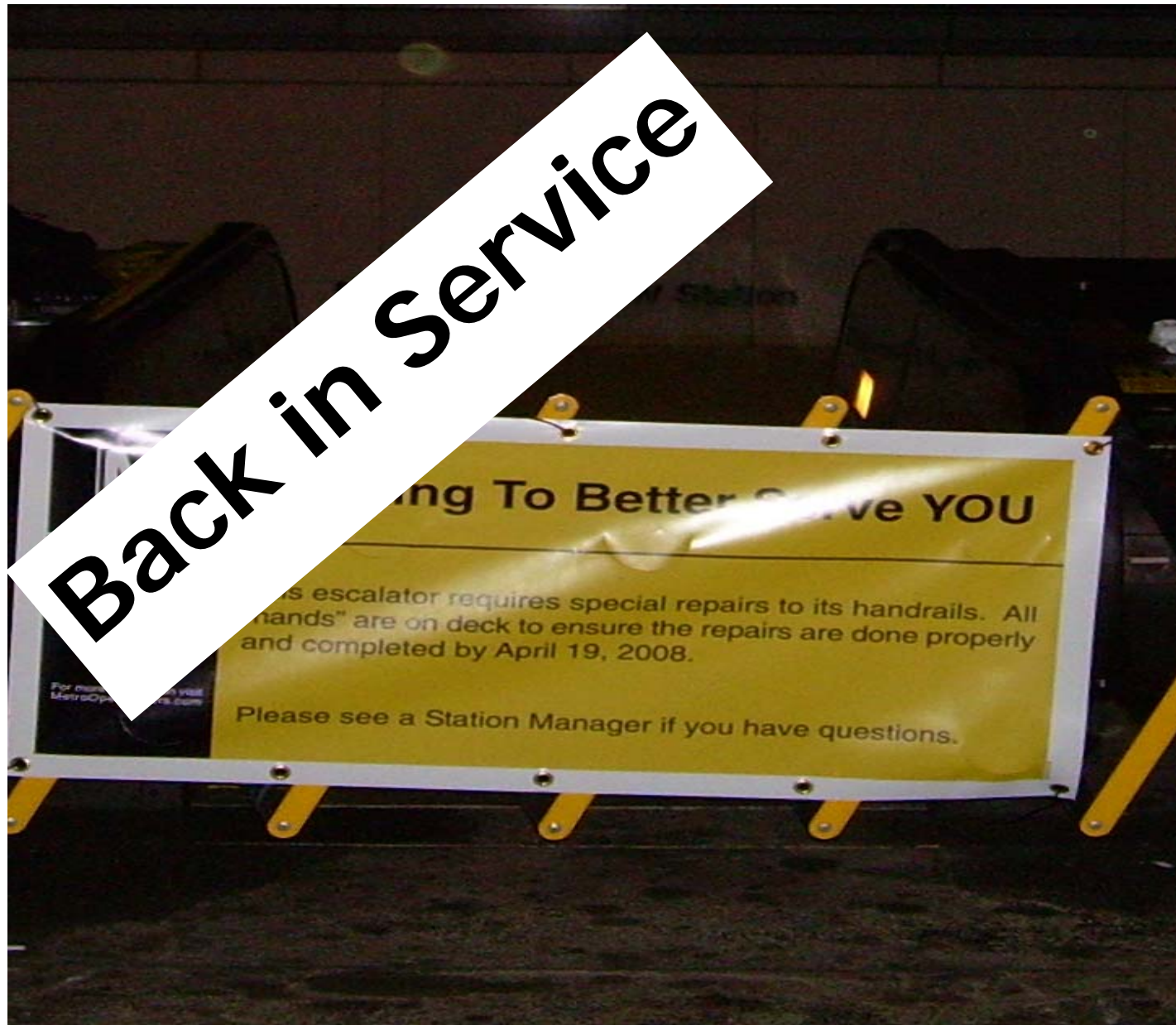
Federal Center SW Escalator – Major Repair
