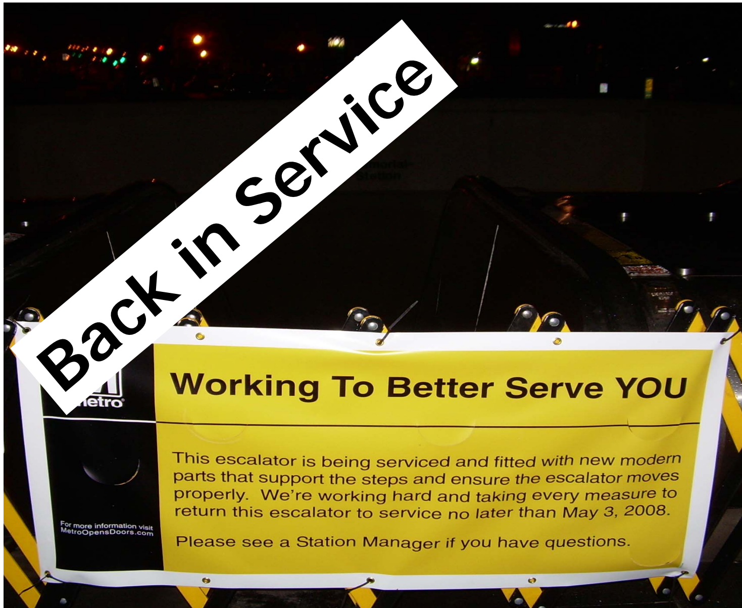
Archives Escalator – Major Repair
