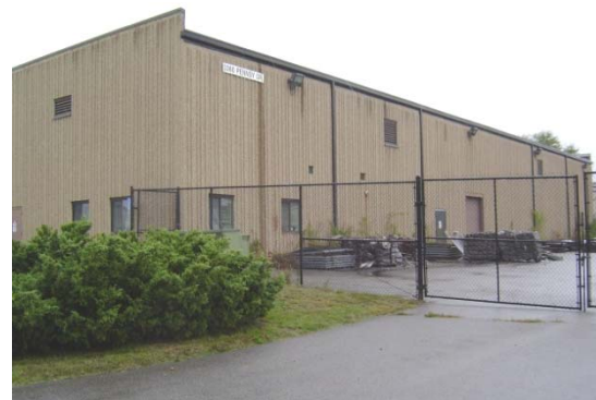
Landover Open Storage Facility
