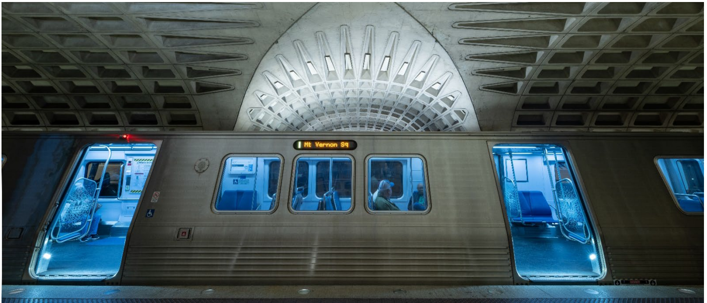
Pictured: Yellow line Metrorail train to Mt. Vernon Square at the L'Enfant Plaza station platform
