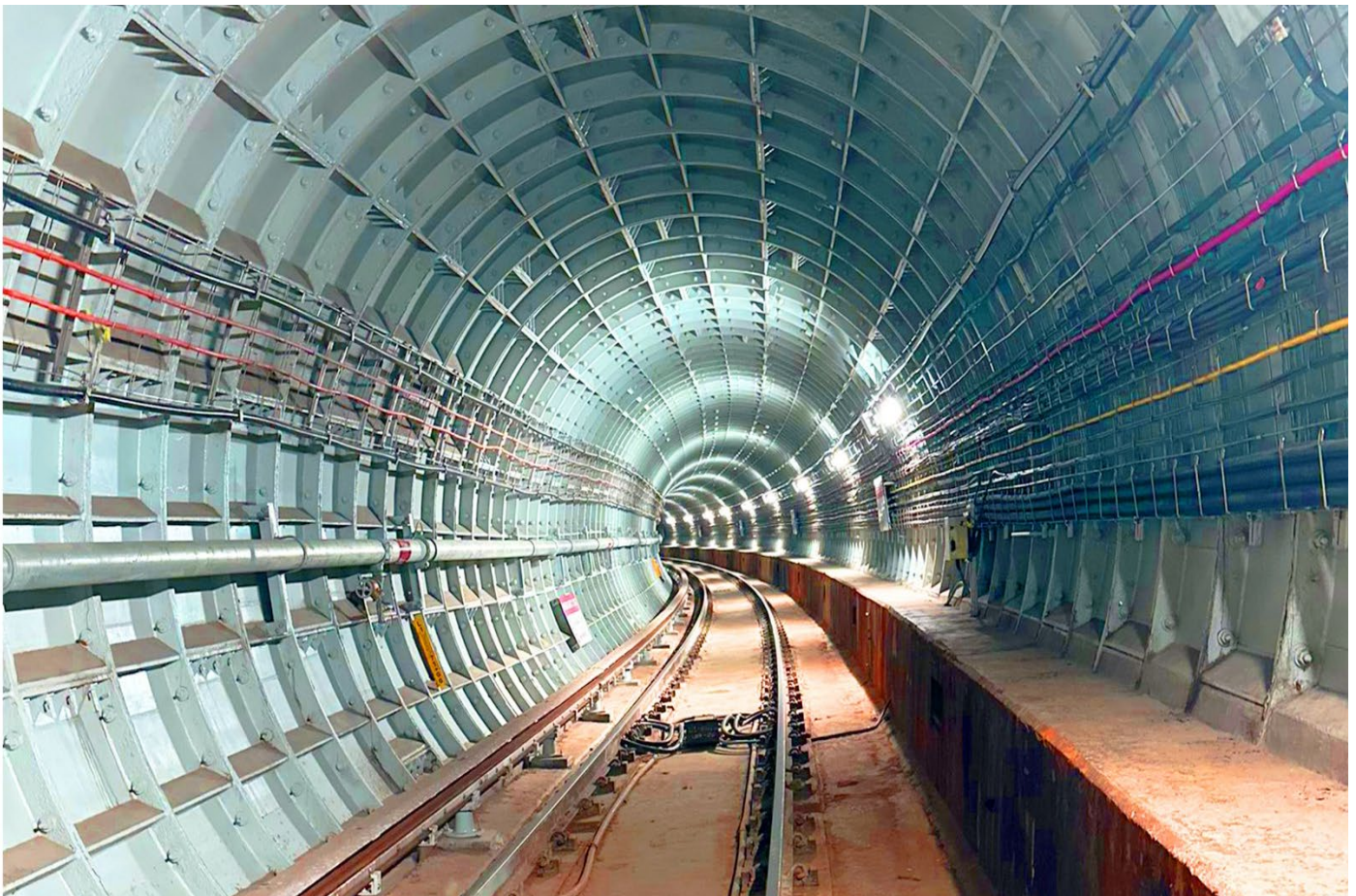
Pictured: Empty underground tunnel and track maintenance of Metro Capital improvement project CIP0349
