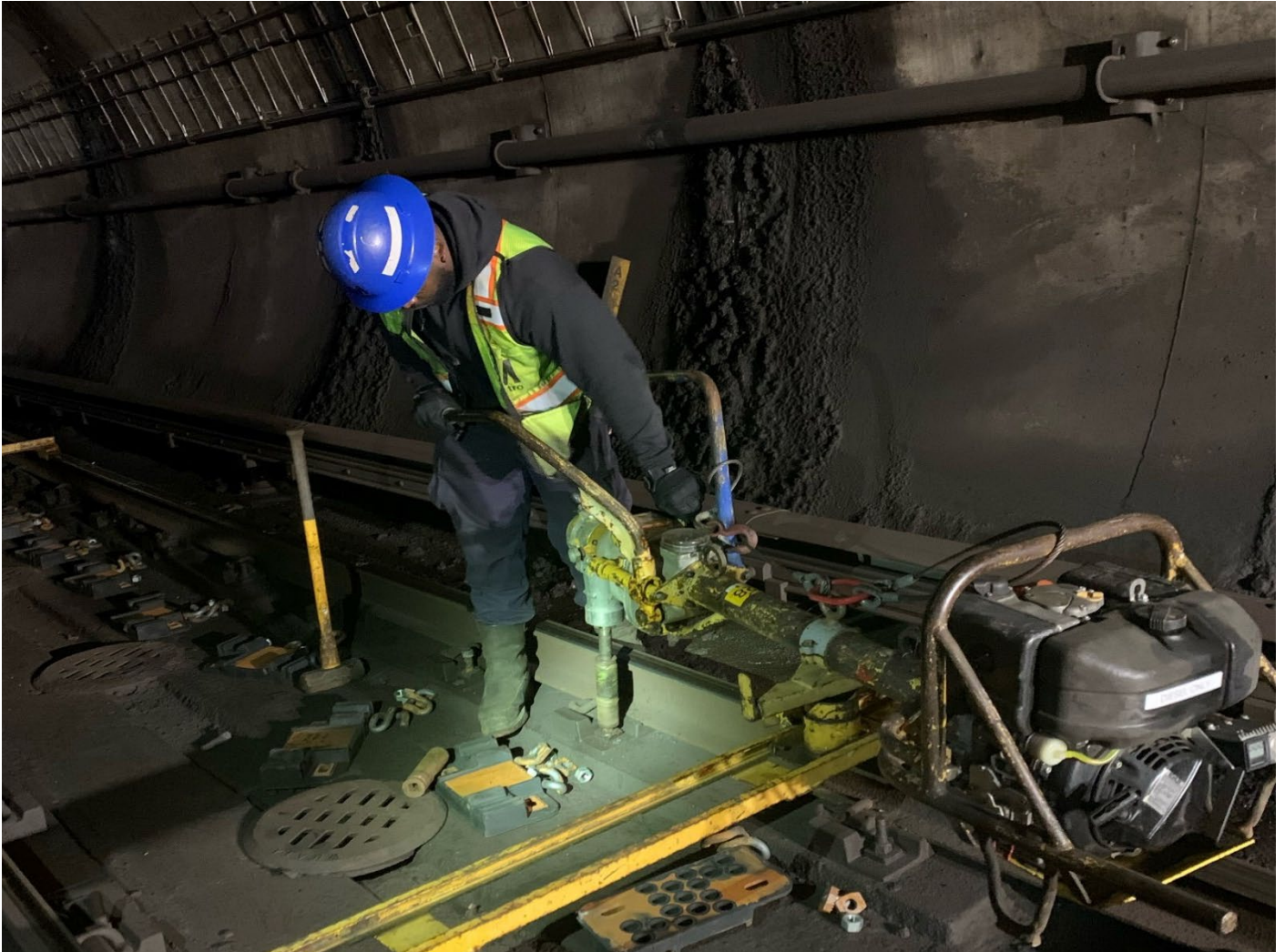
Pictured: Metrorail track maintenance worker in tunnel
