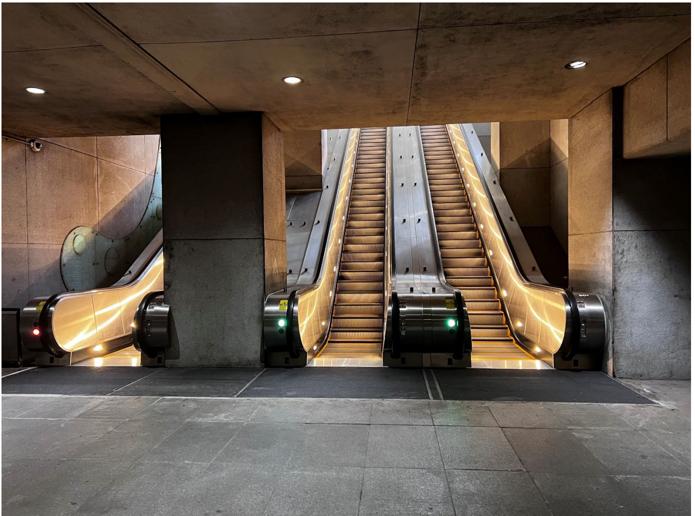
Pictured: Farragut North Escalator Replacement
