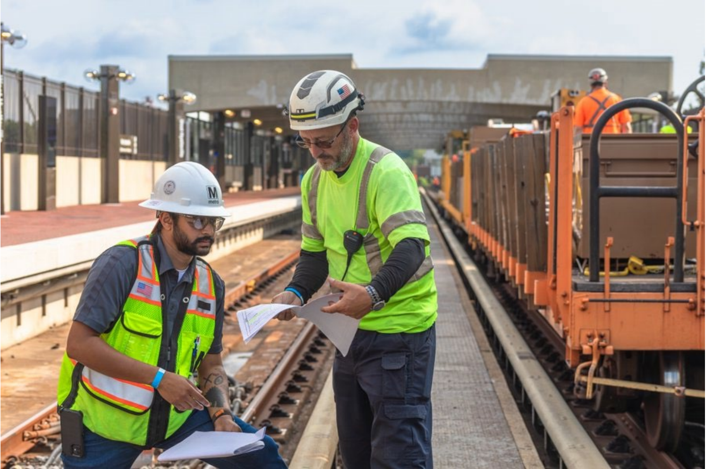
Pictured: Two rail construction workers planning maintenance on station track
