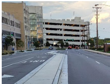
Figure 6: The Metro parking garage as viewed from Halpine Road and Rockville Pike.
